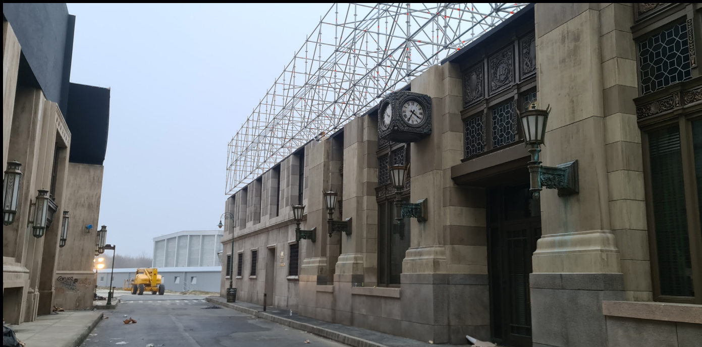
Examples of the scaffold structures used on the Ext Continental and Chinatown sets
