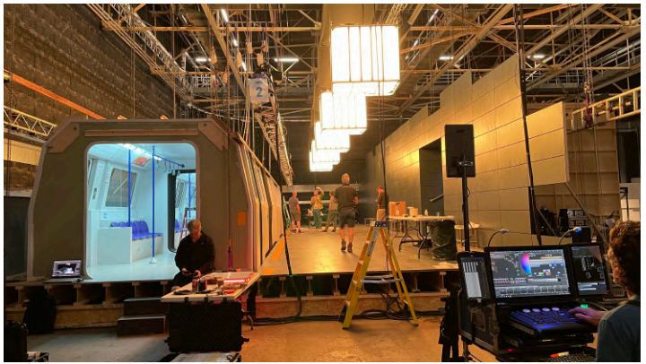
Construction of Subway Train and Platform, front 1/3 of carriage hung on chain tackles to simulate movement between the carriages and scenic painting in the rear set on a sliding rig to give a further perspective shift within the frame
